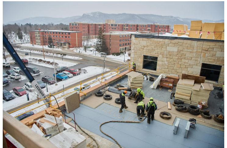
Workers place insulation on the roof of the student center. The building will incorporate a sustainable design strategy with the goal of achieving Leadership in Energy and Environmental Design (LEED) Gold Certification.
