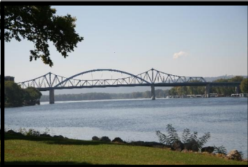
Cass St. Bridge La Crosse, WI
