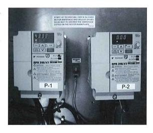
A major benefit of VFDs is their "soft-start" capability that gradually ramps up a motor's operating speed at startup and greatly reduces the stress on components. On typical startup, a constant-speed motor is subject to high torque and electrical surges that can reach up to 10 times the full current load.
