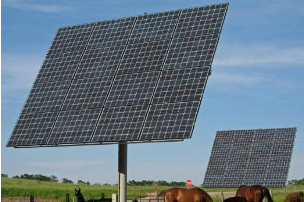
5. Example of a top of pole mounted dual axis tracking PV array. (Photograph H&H Solar Energy Services)
