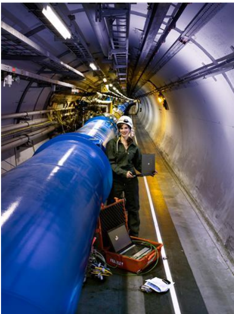
LHC tunnel at CERN
