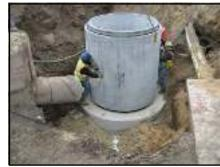
In-Line Stormwater Treatment Device
