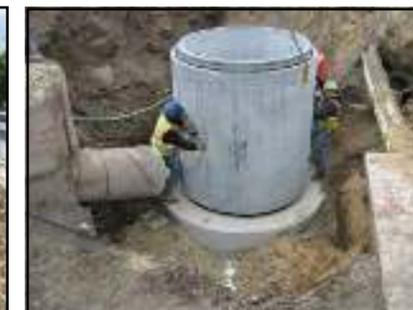
In-Line Stormwater Treatment Device
