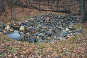
Figure 6.08-3 Field Stone Energy Dissipaters
