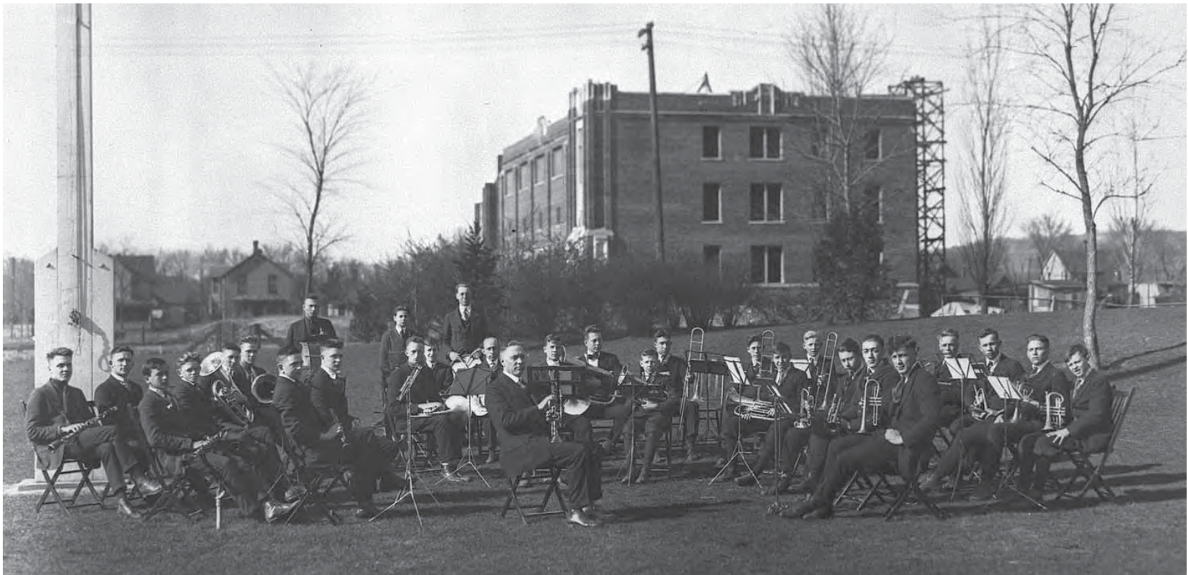
Figure 1.5.6-3: Wittich Hall Under Construction
