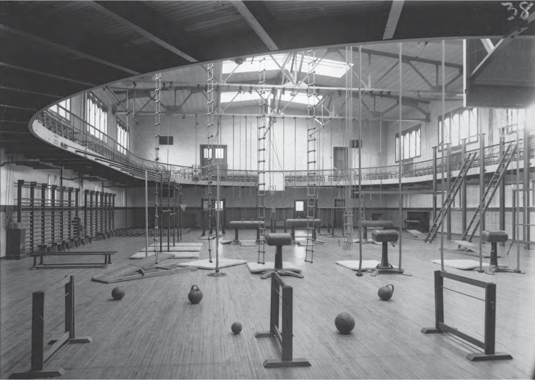
Figure 1.1-1: 1916 Gymnasium; UW-La Crosse Area Research Center (c. 1920)
