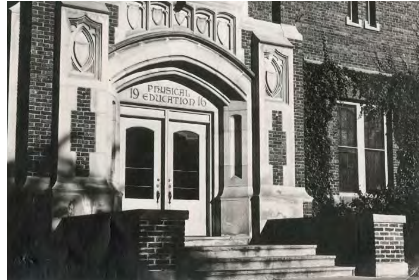
Figure 1.5.6-2: West Elevation; UW–La Crosse Area Research Center (c.1920)
