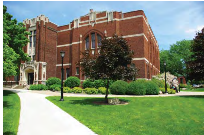
Figure 5.4-1: Existing Exterior – West Elevation
