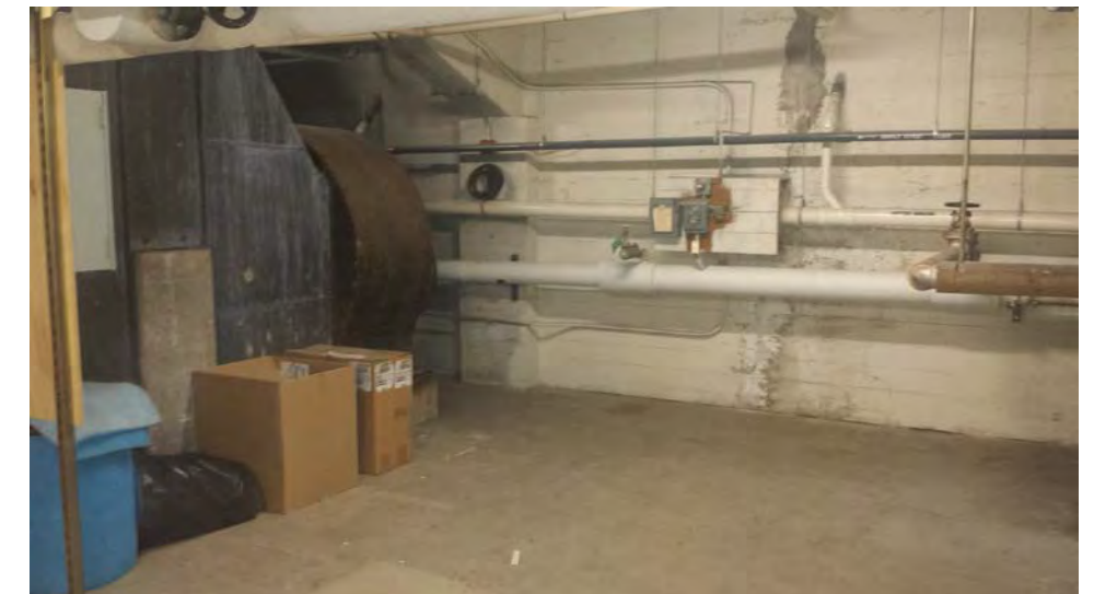
Figure 30: Basement Mechanical Room, Wittich Hall; River Architects (2016)
