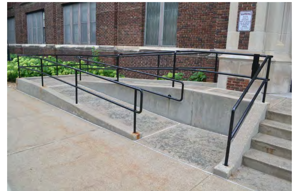
Figure 27: West Ramp, Wittich Hall; River Architects (2016)
