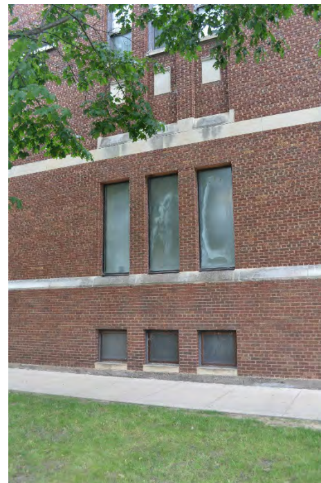
Figure 20: East Elevation, Wittich Hall; River Architects (2016)
