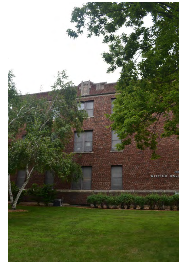
Figure 51: North Elevation, Wittich Hall; River Architects (2016)
