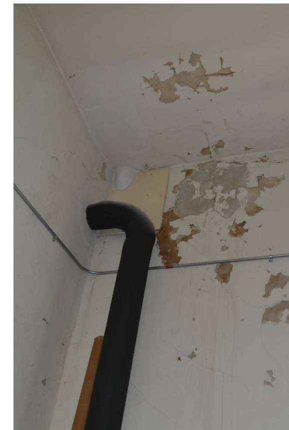
Figure 72: 1916 Gymnasium, Wittich Hall; River Architects (2016)
