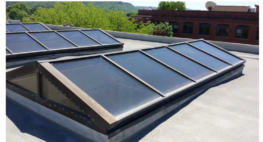
Figure 60: 1930 Skylights, Wittich Hall; River Architects (2014)
