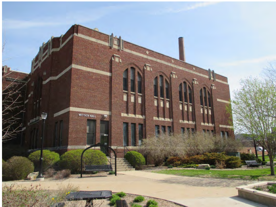
Figure 12: South Elevation, Wittich Hall; River Architects (2014)
