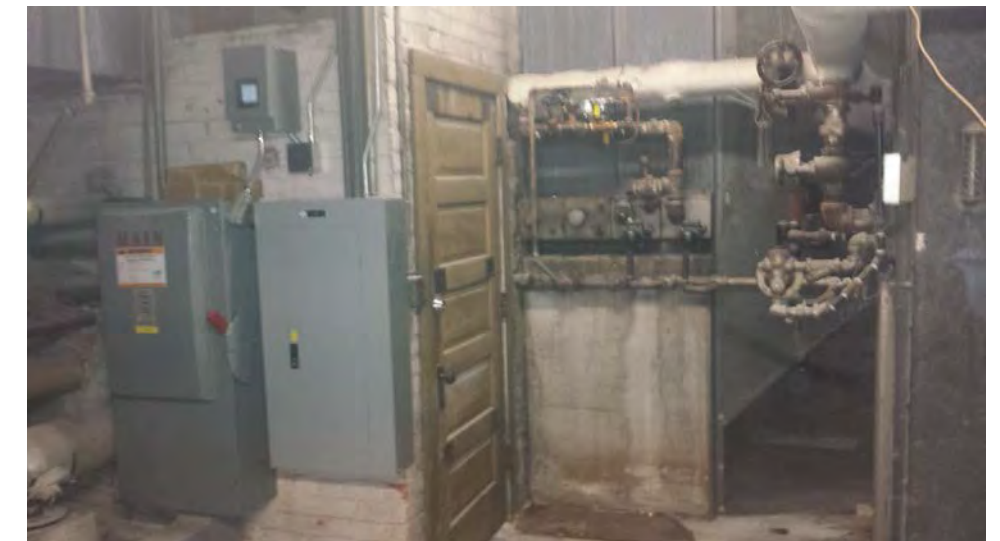
Figure 31: Basement Mechanical Room, Wittich Hall; River Architects (2016)
