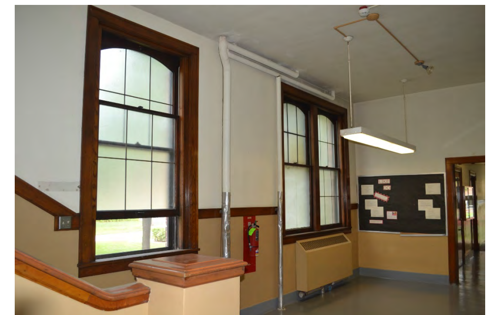
Figure 25: North Entrance Lobby, Wittich Hall; River Architects (2016)
