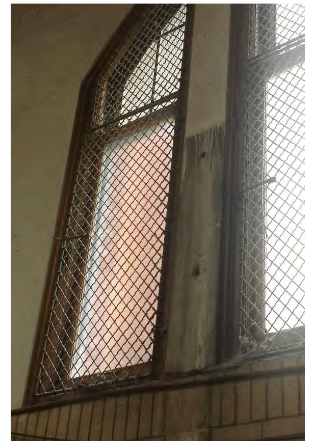
Figure 78: 1930 Gymnasium, Wittich Hall; River Architects (2016)
