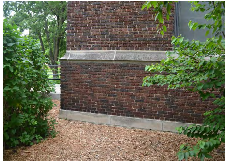
Figure 48: North Elevation, Wittich Hall; River Architects (2016)
