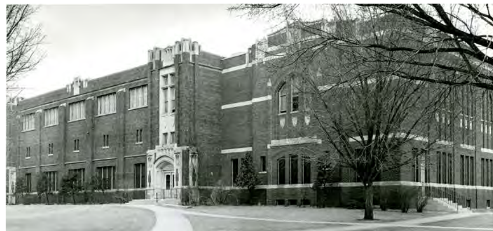
Figure 36: West Elevation, Wittich Hall; UW-La Crosse Area Research Center (c.1940's)
