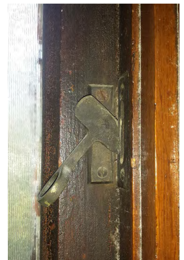
Figure 73: 1916 Gymnasium, Wittich Hall; River Architects (2016)
