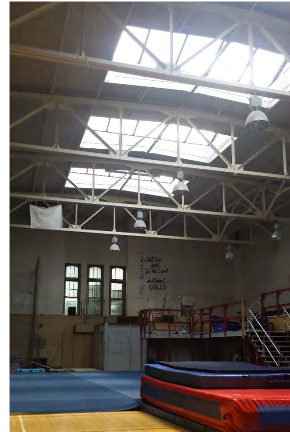
Figure 75: 1930 Gymnasium, Wittich Hall; River Architects (2016)
