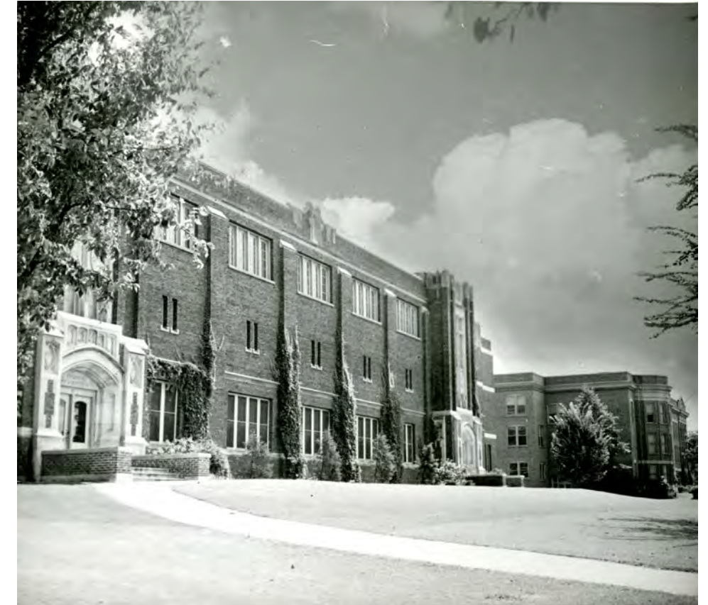
Figure 37: West Elevation, Wittich Hall; UW-La Crosse Area Research Center (c.1930's)
