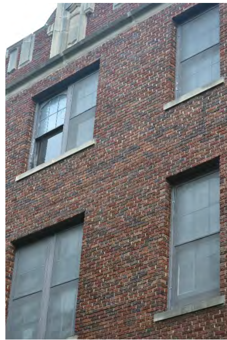
Figure 18: North Elevation, Wittich Hall; River Architects (2016)
