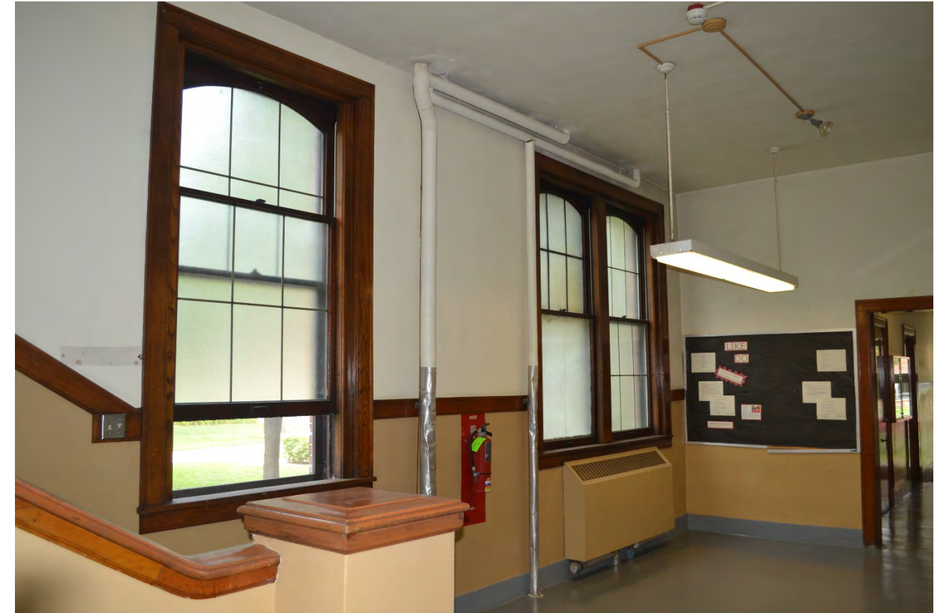
Figure 61: North Entrance Lobby, Wittich Hall; River Architects (2016)
