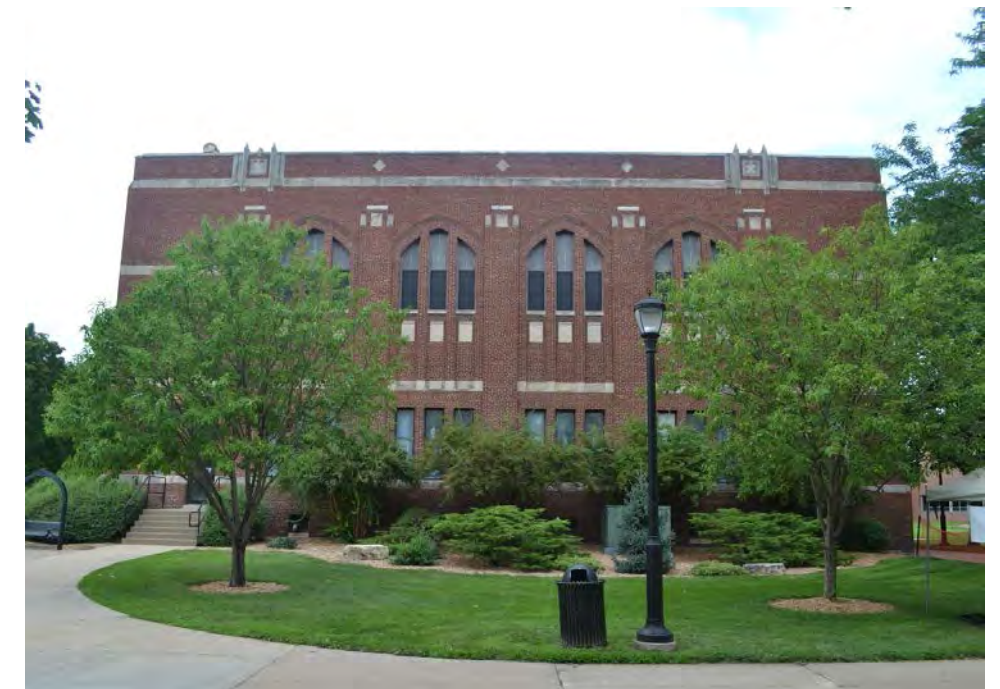
Figure 57: South Elevation, Wittich Hall; River Architects (2016)
