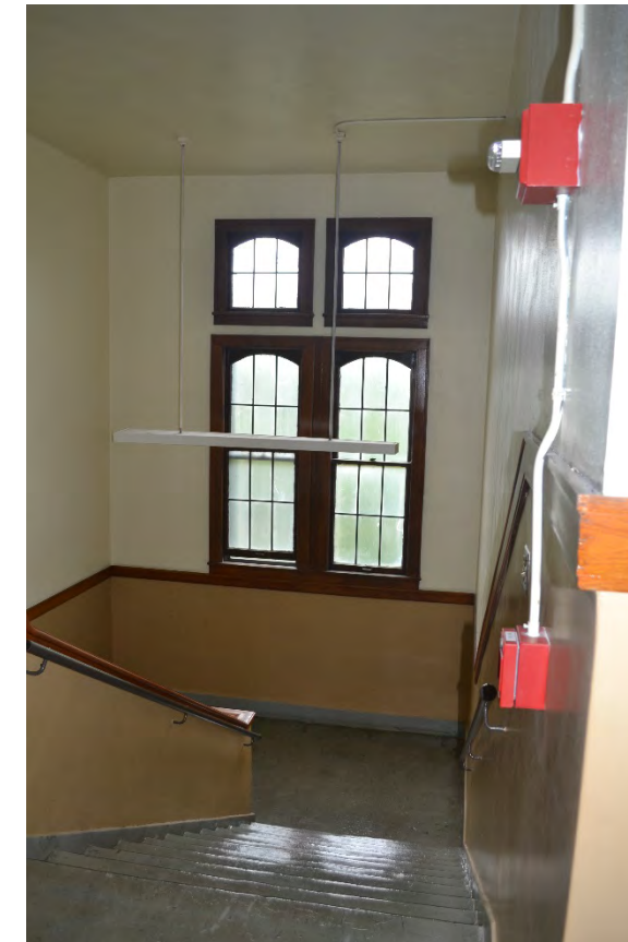
Figure 67: South Entrance Lobby, Wittich Hall; River Architects (2016)
