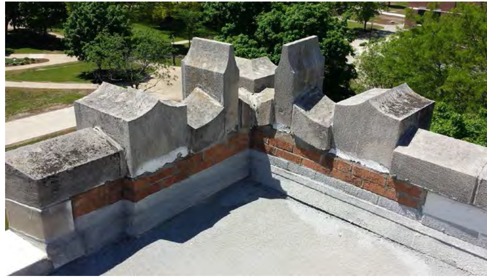
Figure 58: Masonry Parapet, Wittich Hall; River Architects (2014)
