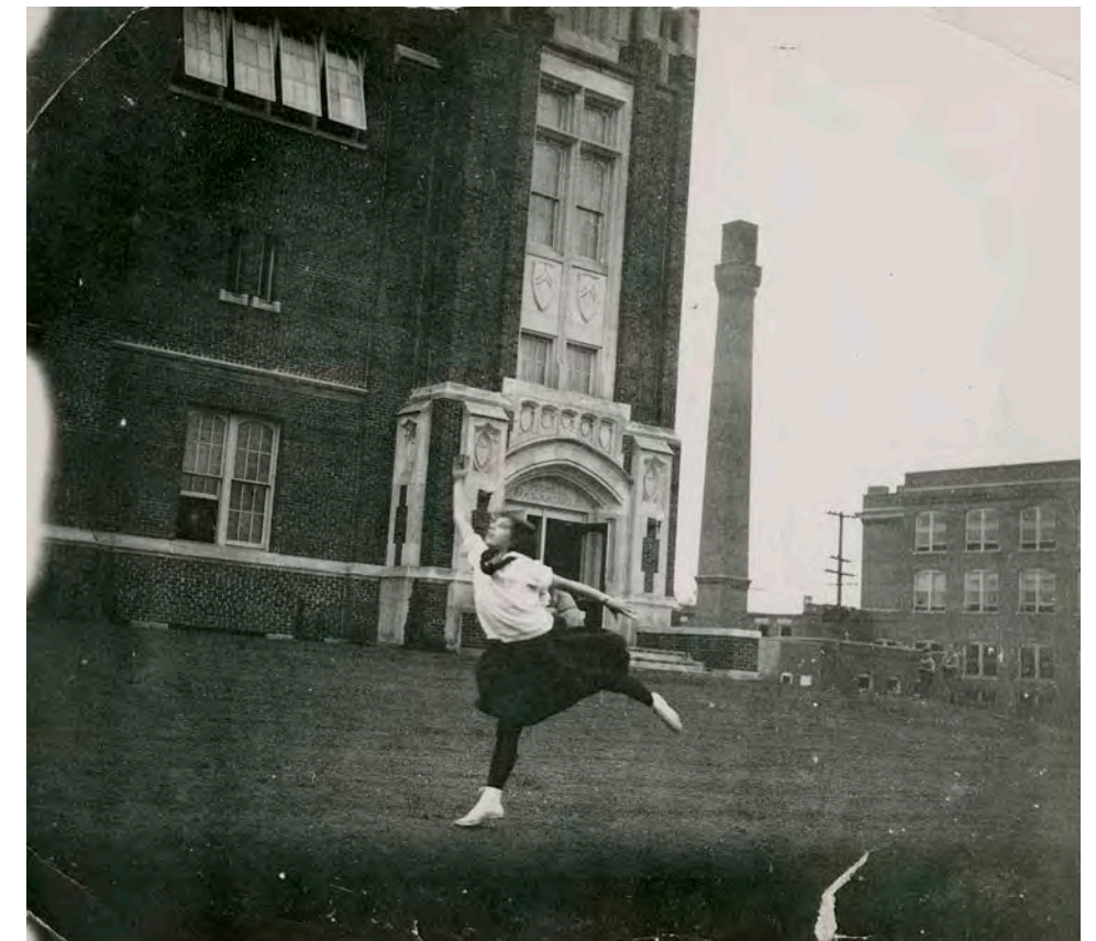
Figure 3: Southwest Entrance, Wittich Hall; UW-La Crosse Area Research Center (c. 1920)
