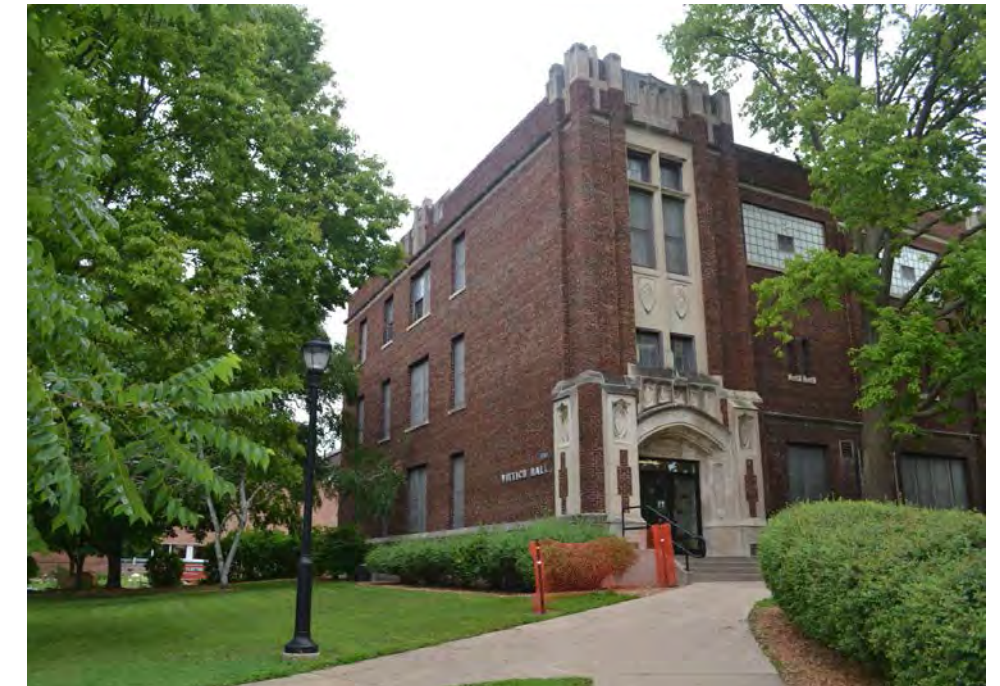
Figure 49: North Elevation, Wittich Hall; River Architects (2016)
