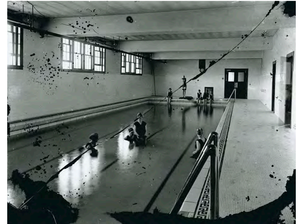
Figure 2: 1916 Pool, Wittich Hall; UW-La Crosse Area Research Center (c. 1920)
