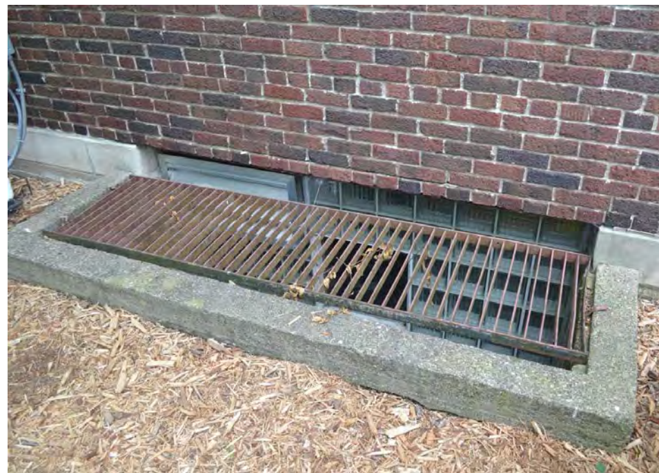
Figure 50: Basement Window, North Elevation, Wittich Hall; River Architects (2016)
