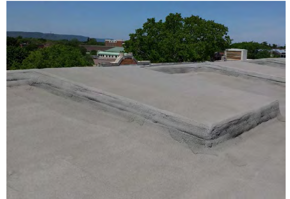
Figure 59: 1916 Skylights, Wittich Hall; River Architects (2014)
