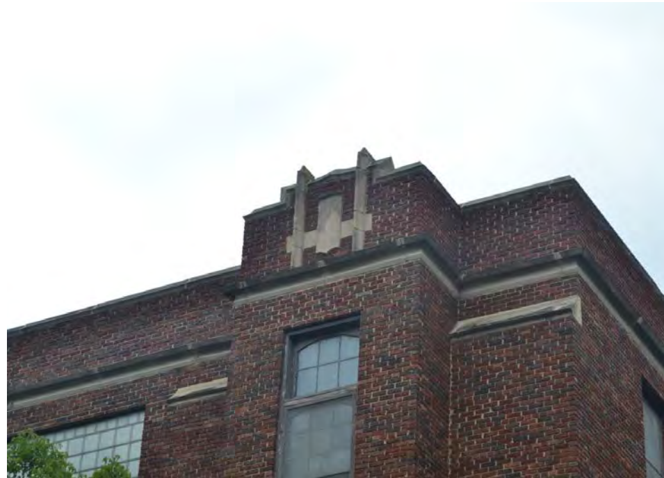
Figure 52: East Elevation, Wittich Hall; River Architects (2016)
