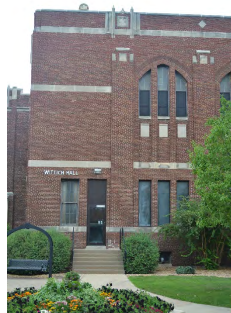
Figure 21: South Elevation, Wittich Hall; River Architects (2016)
