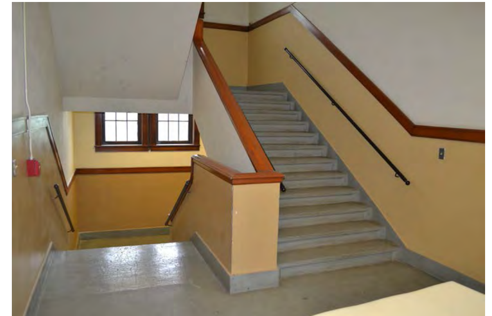
Figure 26: Typical Stair, Wittich Hall; River Architects (2016)
