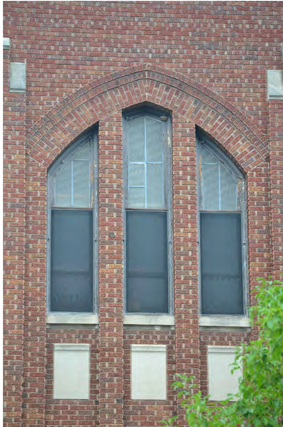
Figure 55: South Elevation, Wittich Hall; River Architects (2016)
