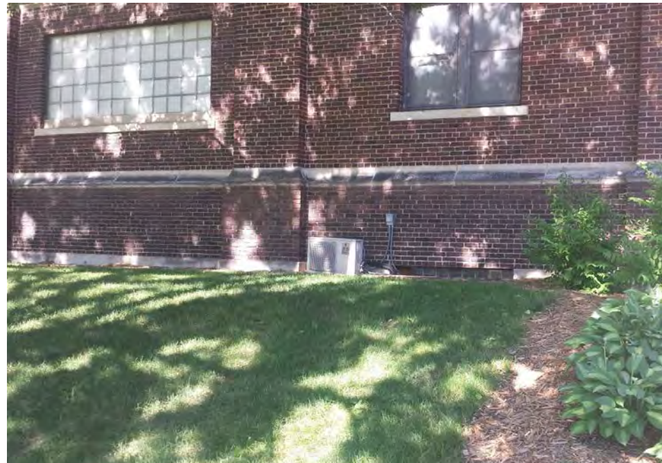
Figure 53: East Elevation, Wittich Hall; River Architects (2016)
