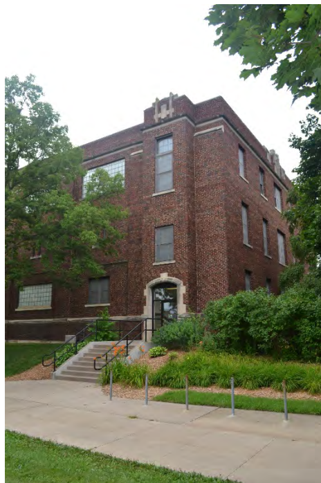
Figure 19: East Elevation, Wittich Hall; River Architects (2016)
