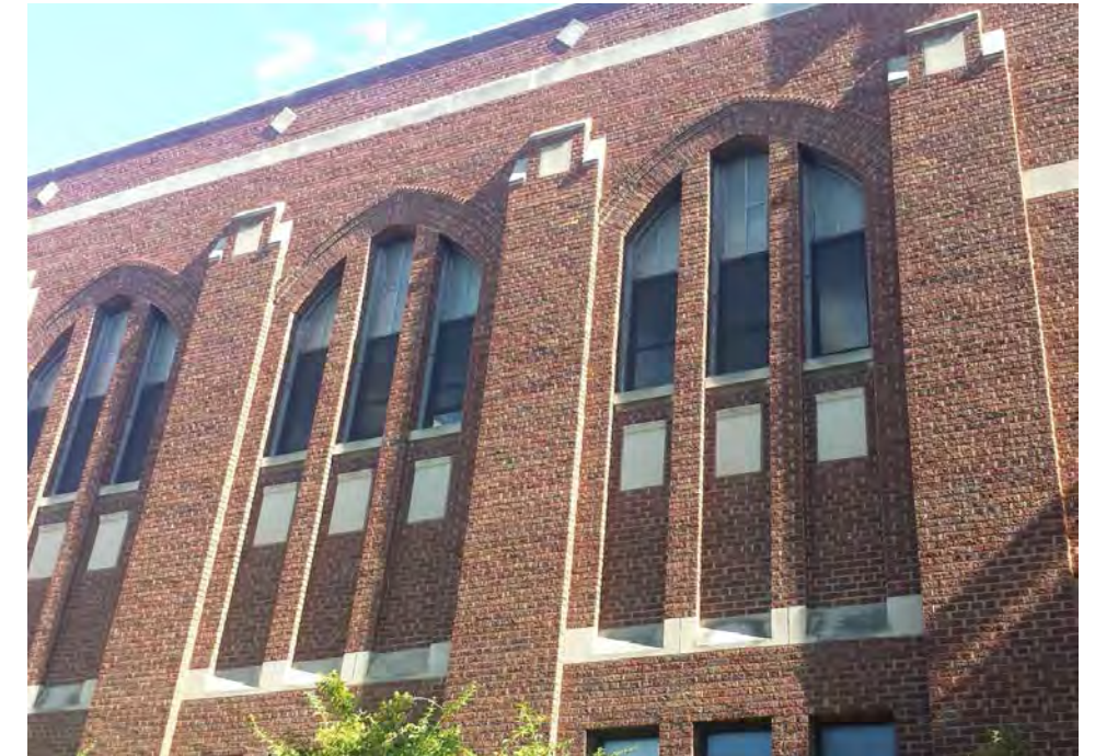
Figure 56: South Elevation, Wittich Hall; River Architects (2016)
