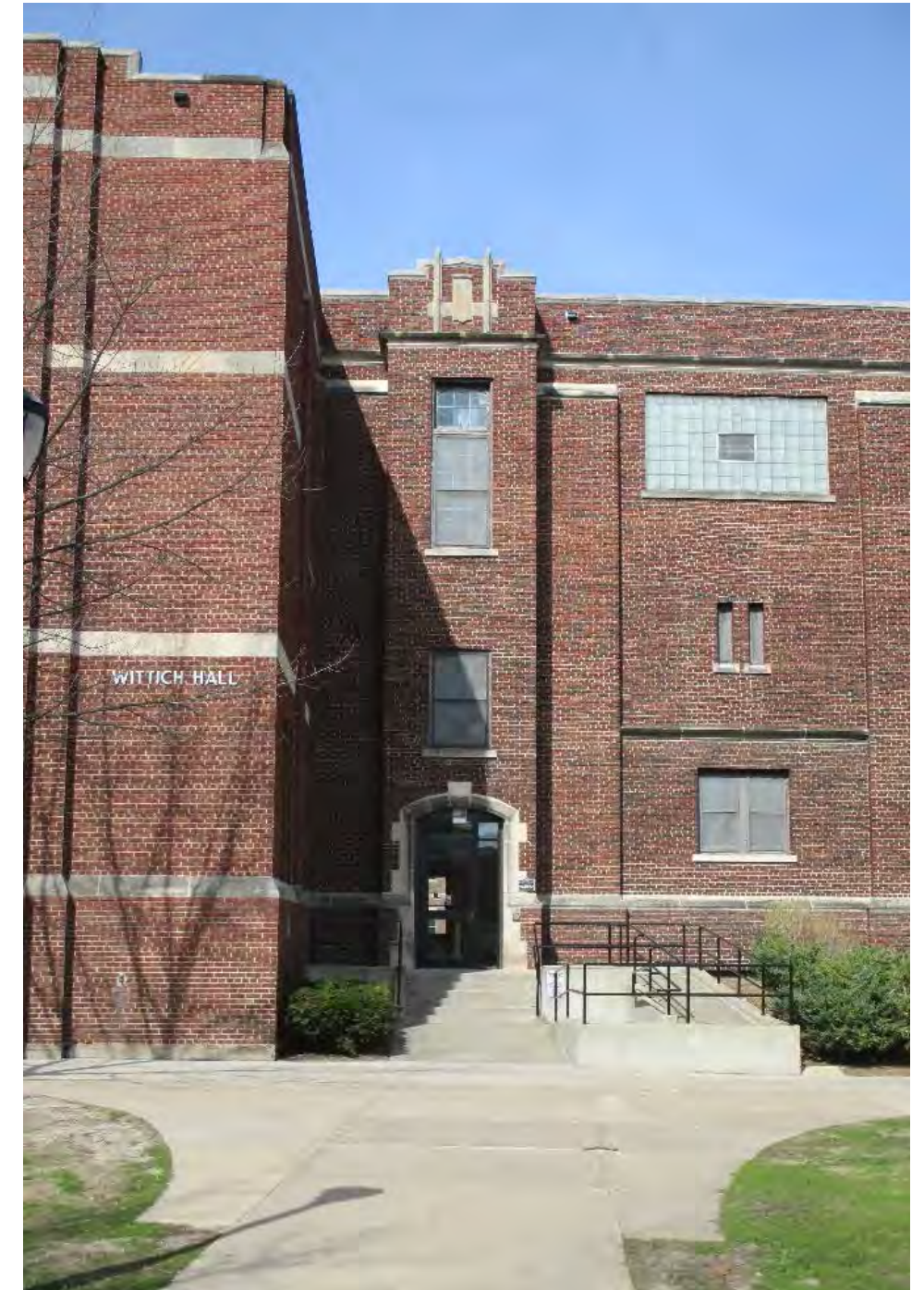
Figure 54: East Elevation, Wittich Hall; River Architects (2016)
