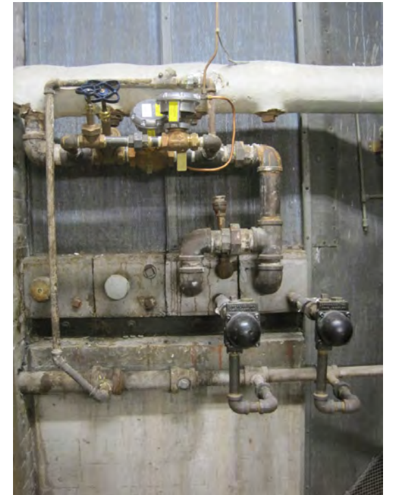
M-17-STEAM HEATING COIL
