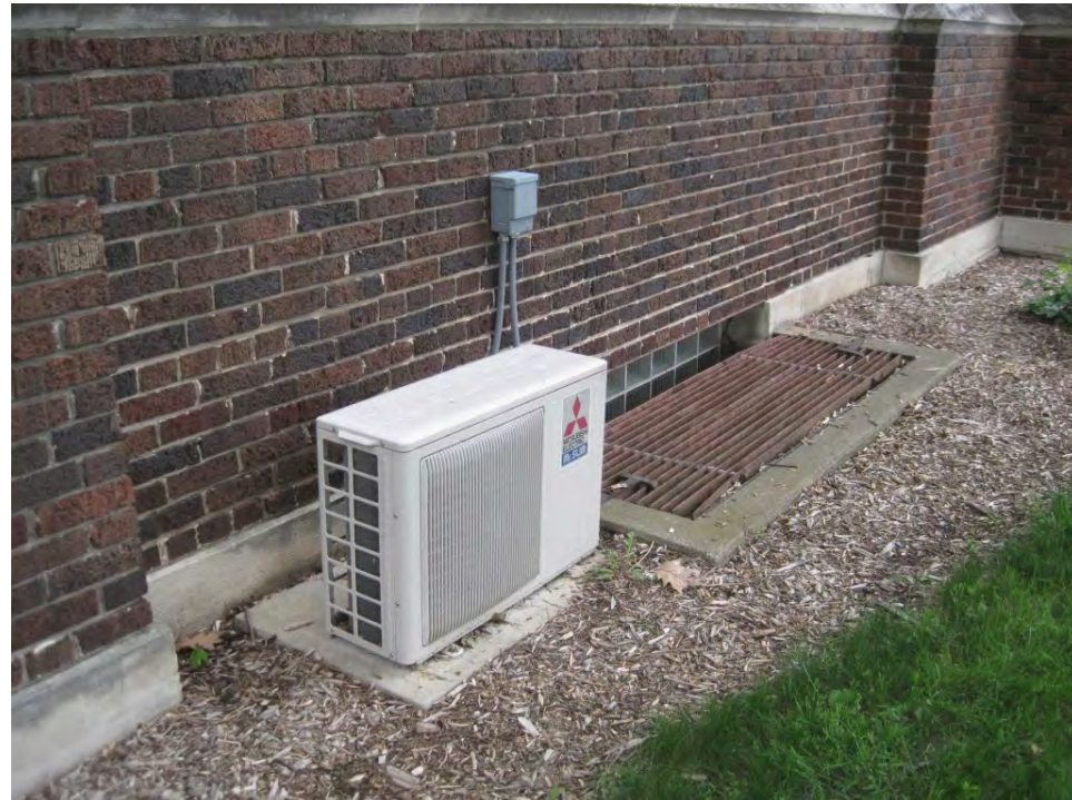
M-09-CONDENSING ACCU-1
