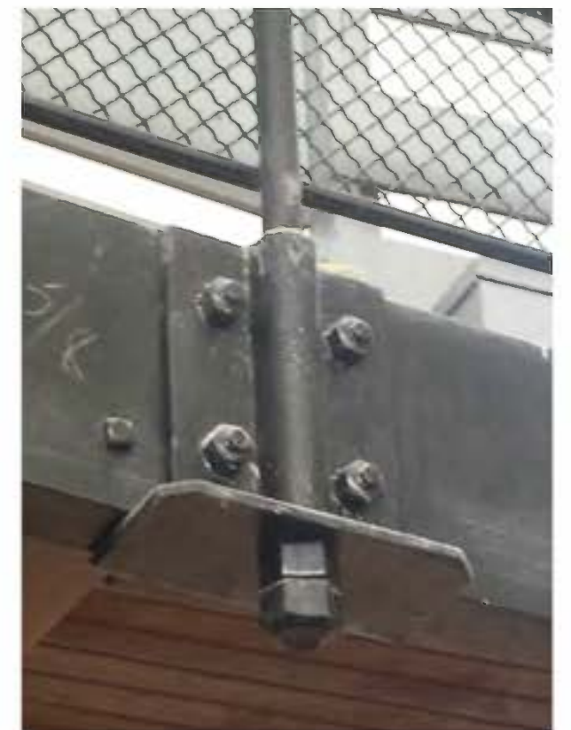
Figure 75: 1916 Gymnasium Suspension Rod, Wittich Hall; River Architects (2016)
