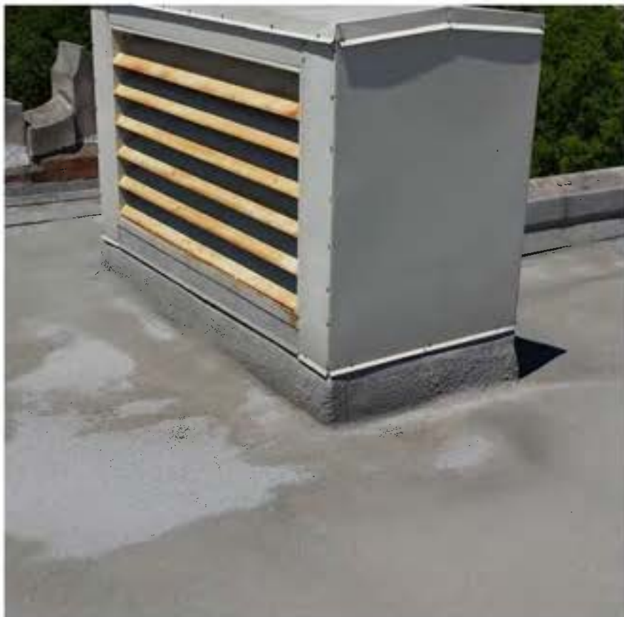
Figure 49: Roof-Top Mechanical Equipment, Wittich Hall: River Architects (2014)
