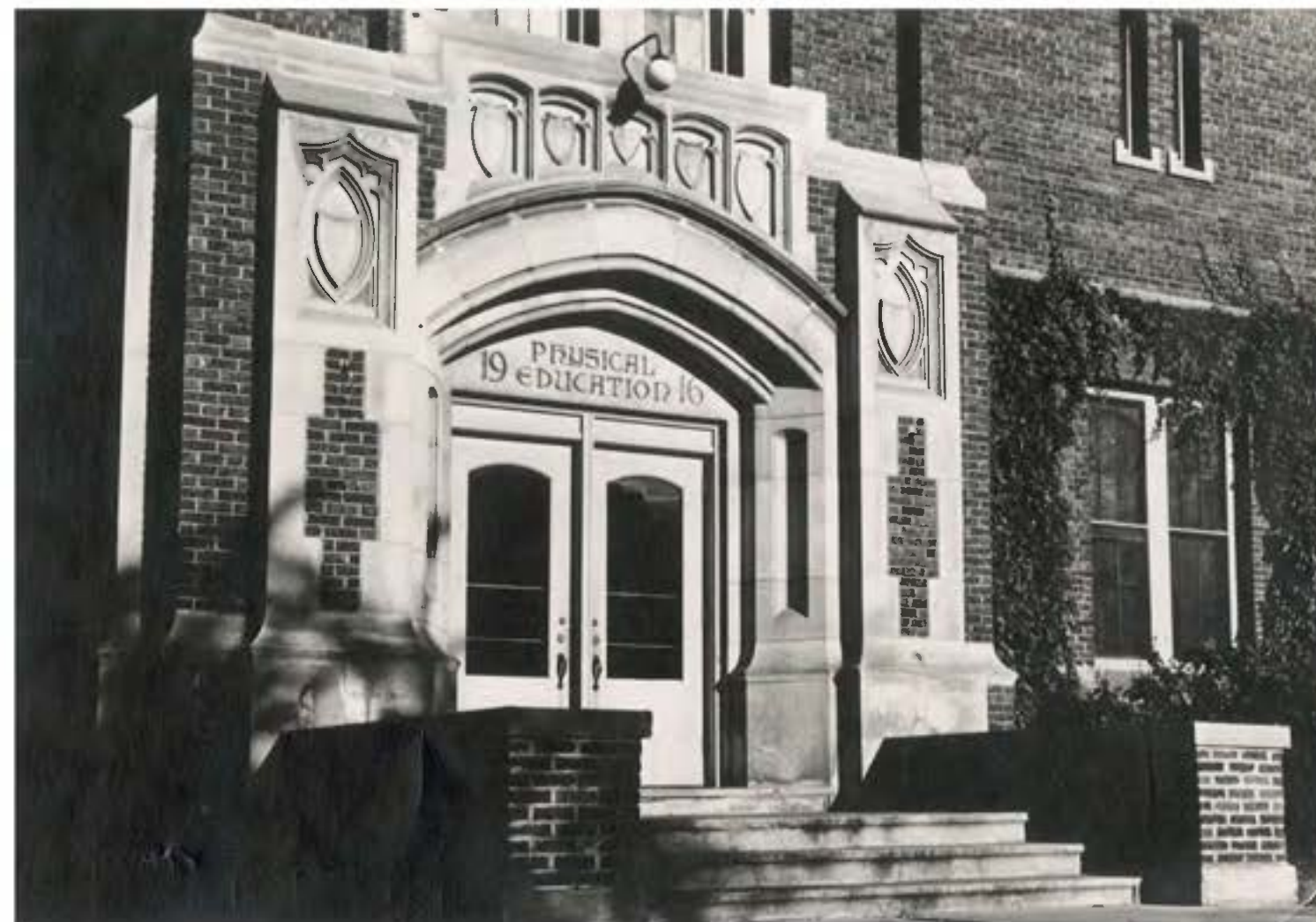
Figure 22: Northwest Entrance, Wittich Hall; UW-La Crosse Area Research Center (c.1920)
