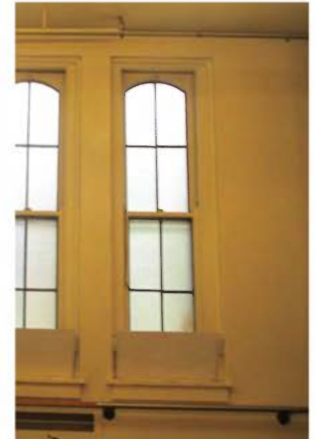
Figure 89: Women’s Locker Room Windows, Wittich Hall; River Architects (2016)
