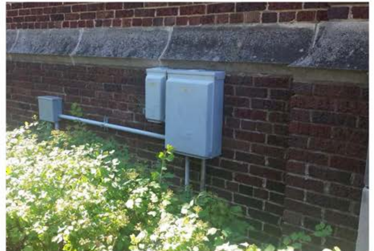
Figure 34: Electrical Equipment, Wittich Hall: River Architects (2016)
