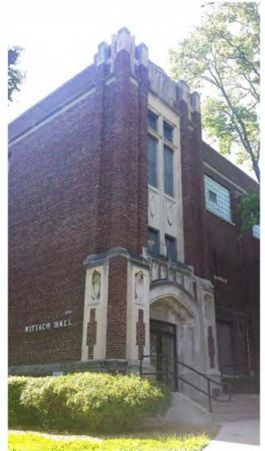
Figure 3: Northwest Entrance, Wittich Hall; River Architects (2016)
