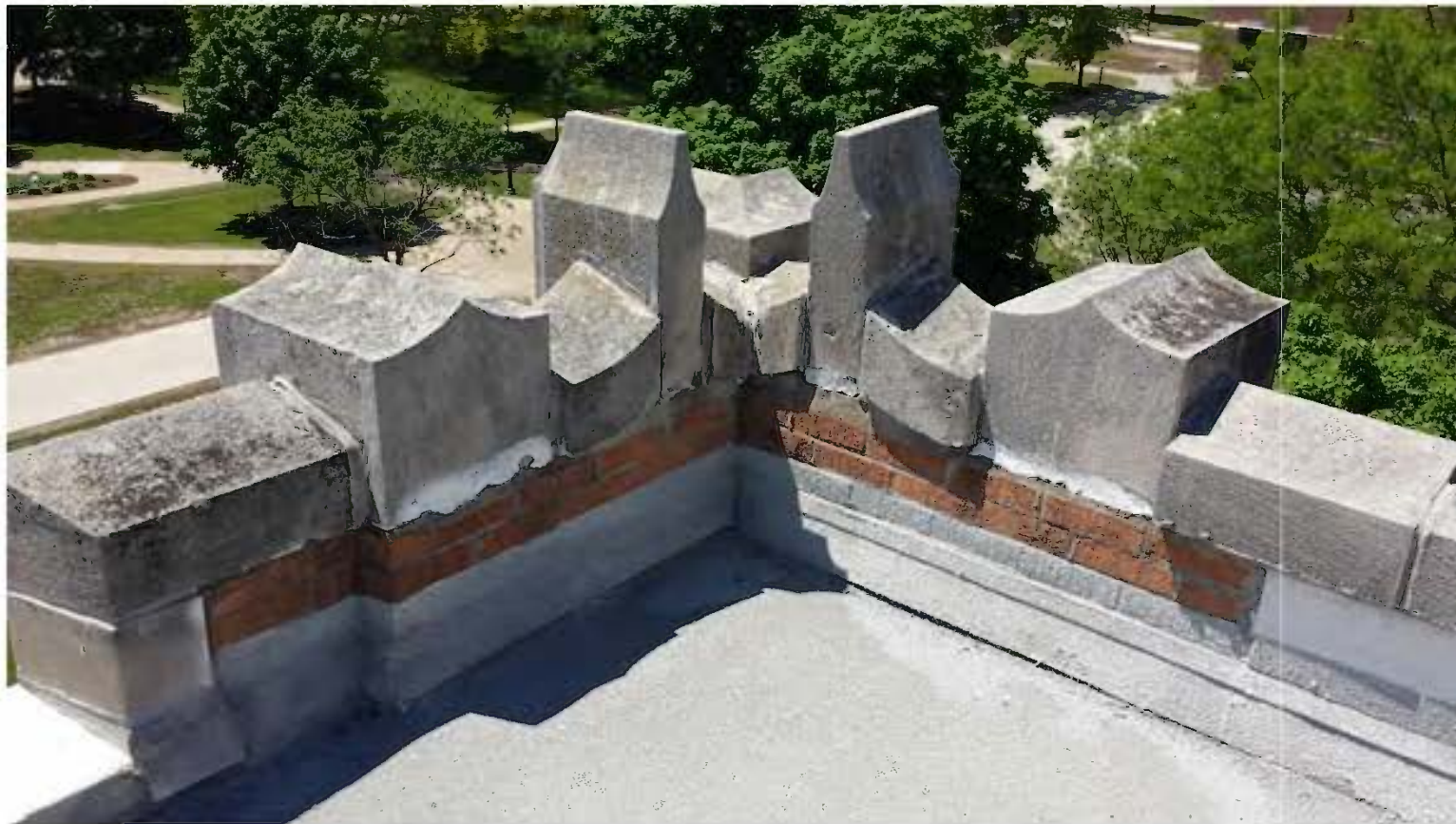
Figure 46: Limestone Copings, Wittich Hall: River Architects (2014)
