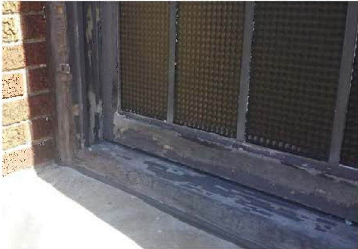
Figure 44: South Window, Wittich Hall: River Architects (2016)
