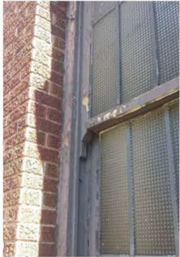
Figure 45: South Window, Wittich Hall: River Architects (2016)
