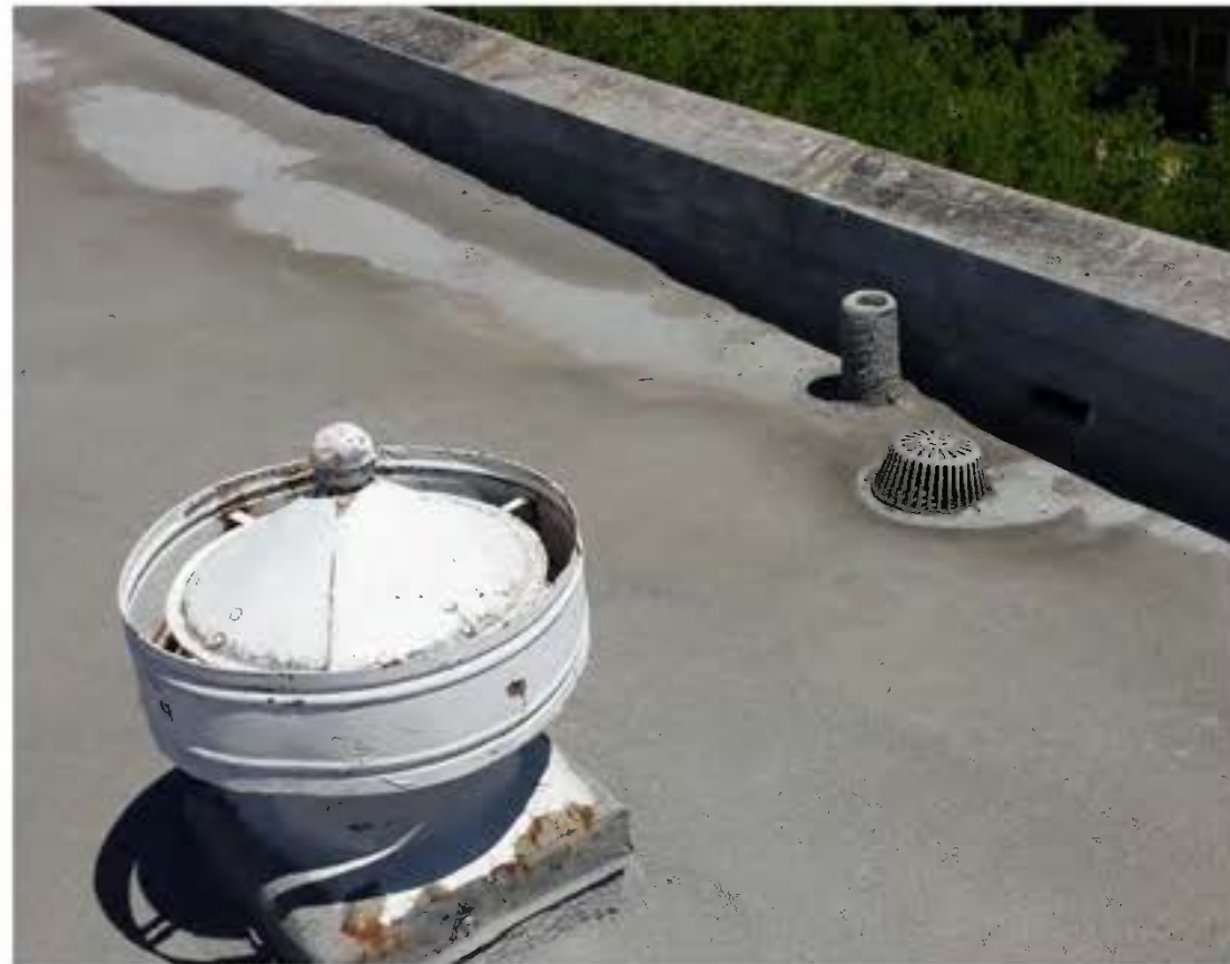
Figure 50: Roof-Top Ventilation Equipment, Wittich Hall: River Architects (2014)
