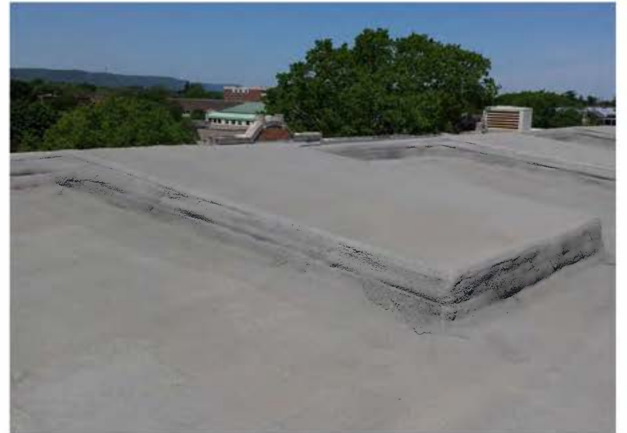
Figure 47: 1916 Skylights with Hypalon Roof Coating, Wittich Hall: River Architects (2014)
