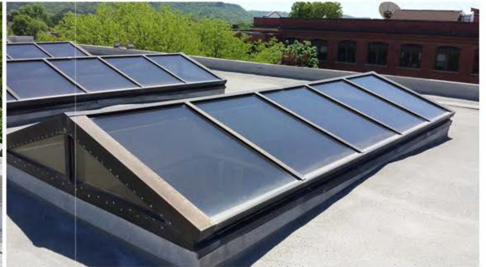
Figure 48: 1930 Addition, Replaced Skylights, Wittich Hall: River Architects (2014)
