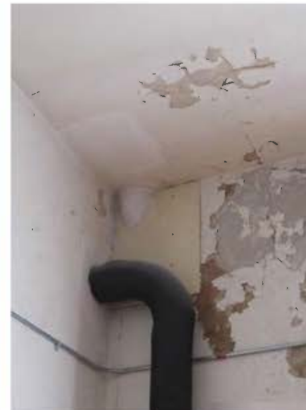
Figure 74: 1916 Gymnasium Roof Drain, Wittich Hall; River Architects (2014)
