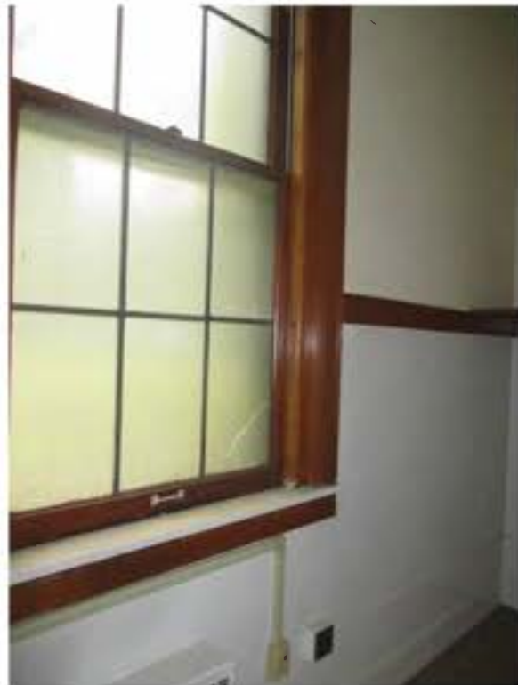
Figure 57: Storage Room 107, Wittich Hall; River Architects (2016)
