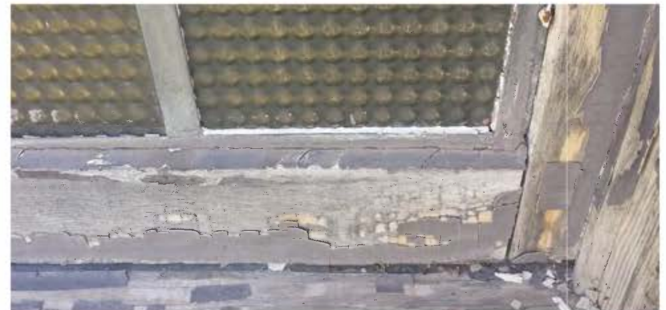
Figure 98: Window Sash, Wittich Hall: River Architects (2016)
