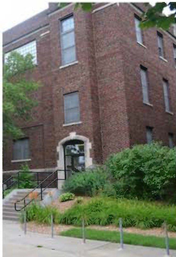
Figure 37: Southeast Entrance, Wittich Hall: River Architects (2016)
