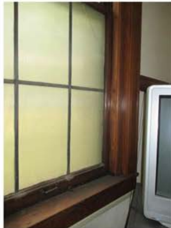
Figure 59: Storage Room 106, Wittich Hall; River Architects (2016)
