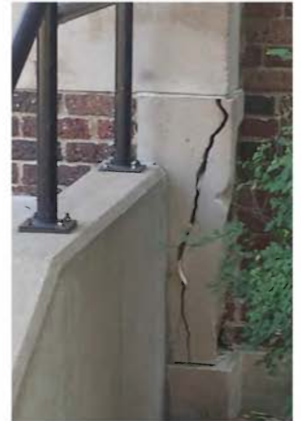
Figure 26: Northwest Entrance, Wittich Hall: River Architects (2016)
