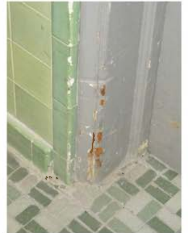
Figure 83: 1930 Pool Door Jamb, Wittich Hall; River Architects (2016)
