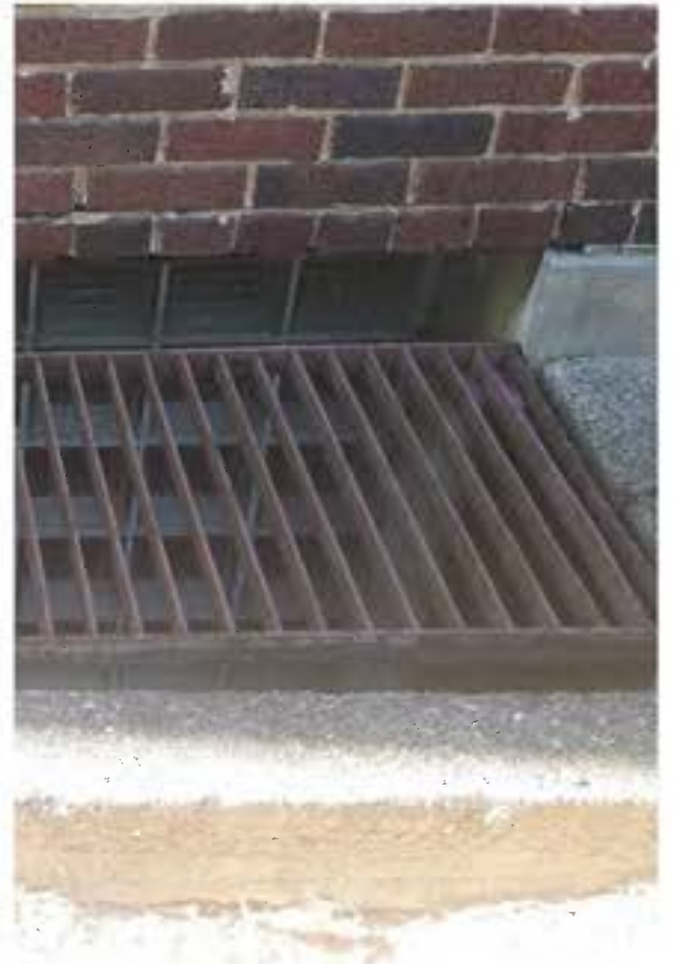
Figure 32: North Window Well, Wittich Hall: River Architects (2016)
