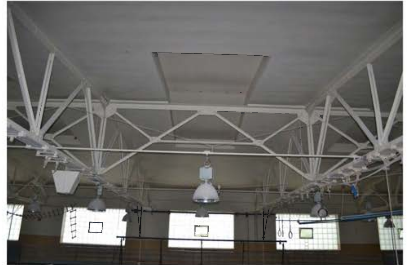
Figure 94: 1916 Gymnasium Roof Structure, Wittich Hall; River Architects (2016)
