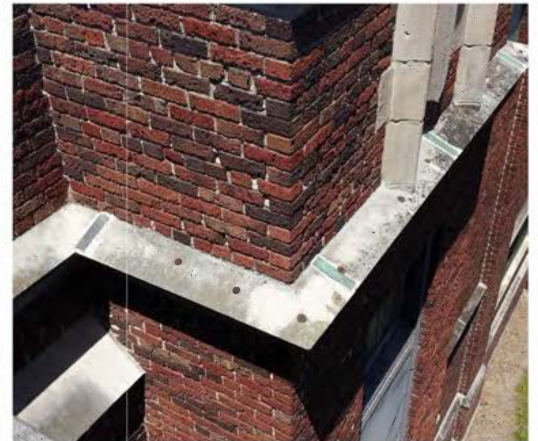
Figure 51: Stone Cornice Flashing Strip, Wittich Hall: River Architects (2014)
