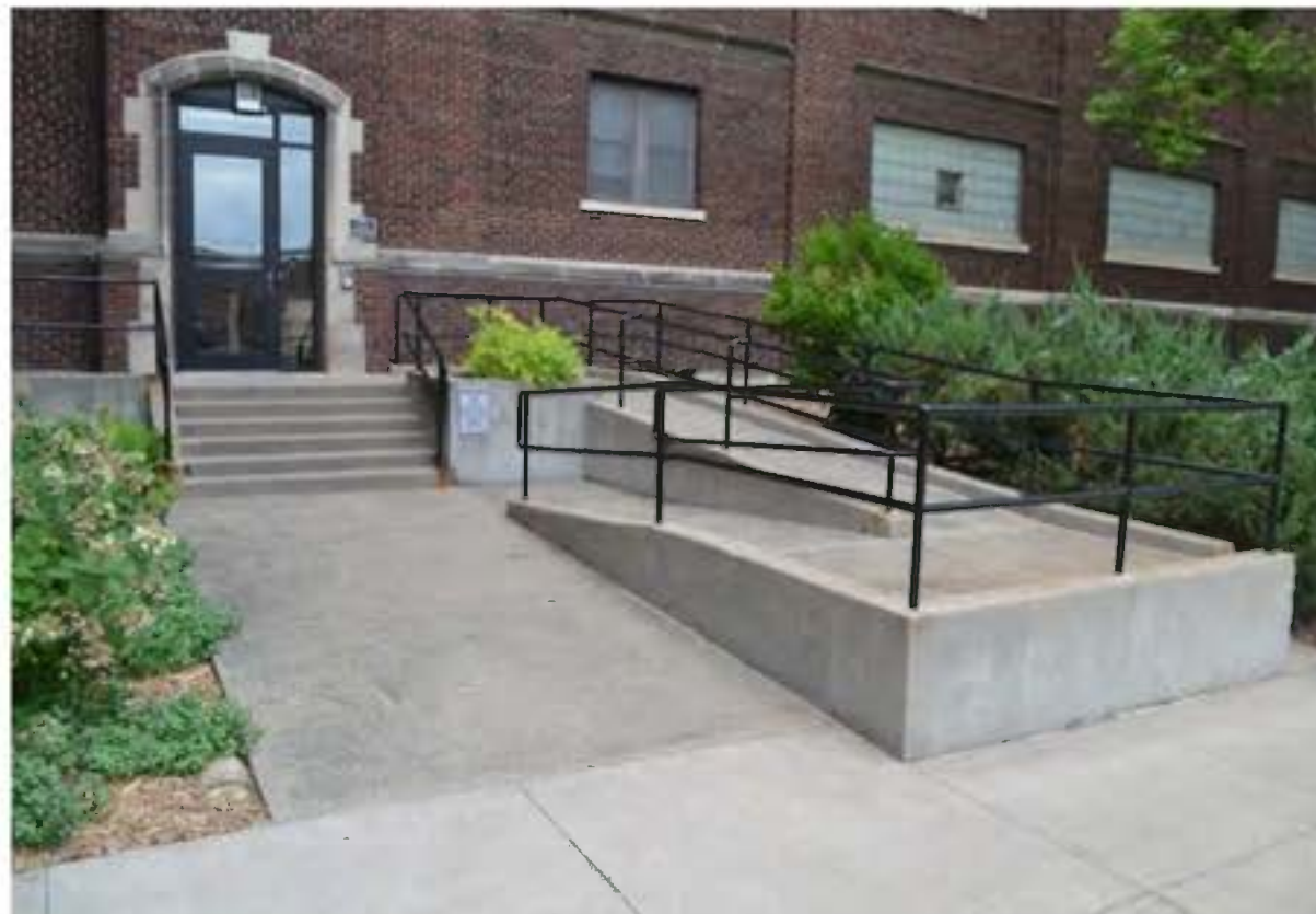
Figure 38: Southeast Entrance, Wittich Hall: River Architects (2016)
