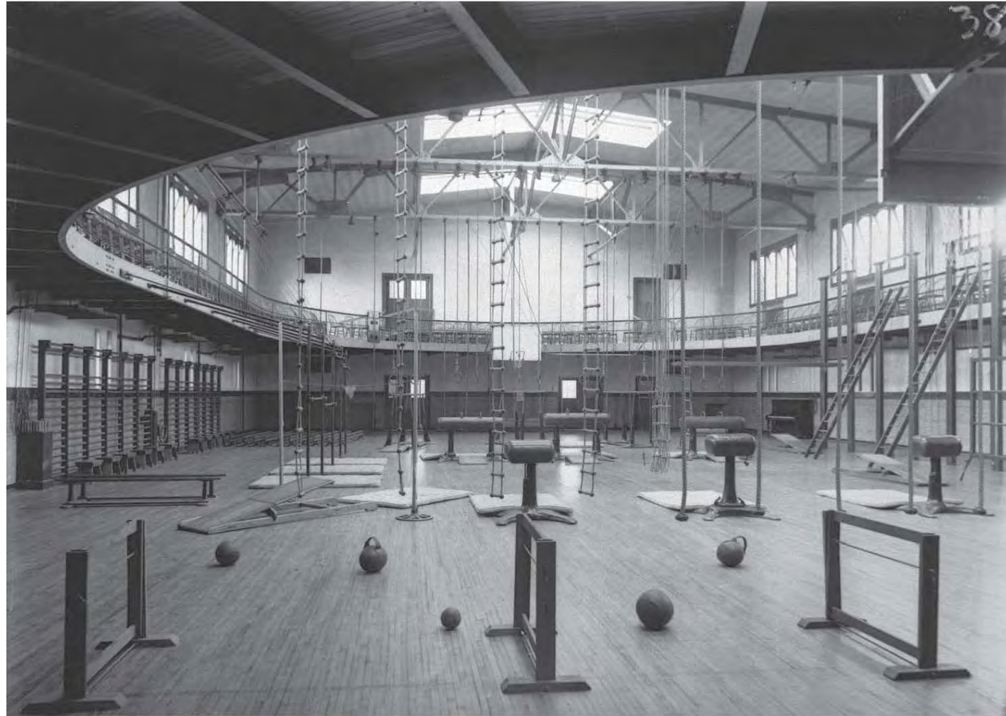
Figure 1.1-1: 1916 Gymnasium; UW-La Crosse Area Research Center (c. 1920)
