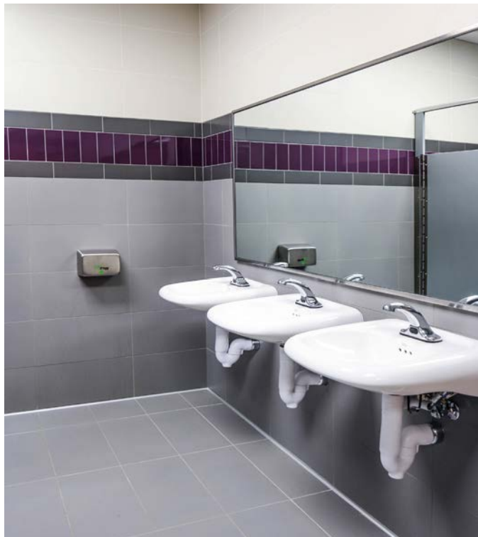
Example of new restroom
