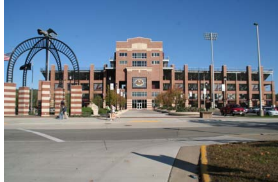
Veterans Memorial Sports Field Complex Completed 2009
