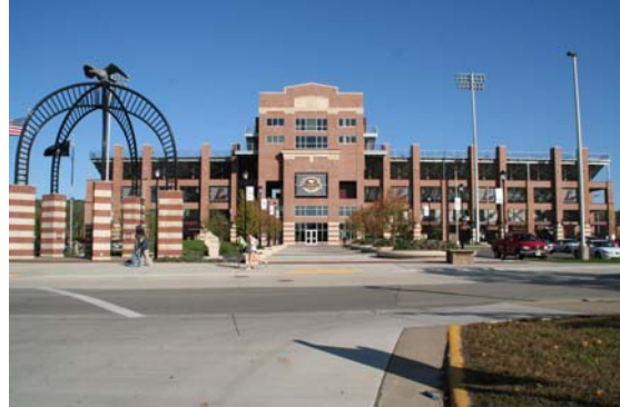
Veterans Memorial Sports Field Complex Completed 2009
