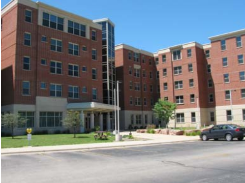
Reuter Hall – Completed 2006
