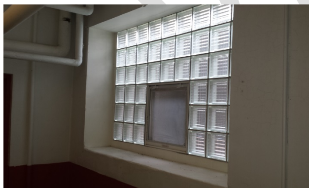
Level 0 Window – 1916 Wing (2014)
