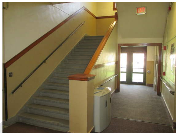
Northwest Interior Stair (2014)
