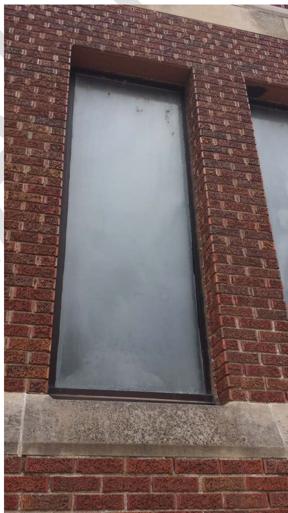
Level 1 Pool Window – 1930 Wing (2014)
