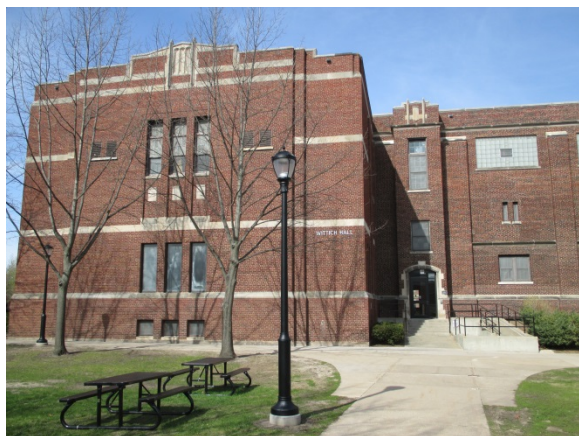
East Elevation – 1930 Addition (2014)
