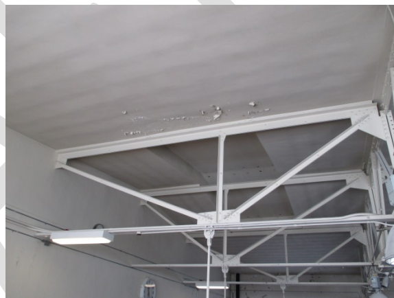
Gymnasium Roof Truss – 1916 Wing (2014)
