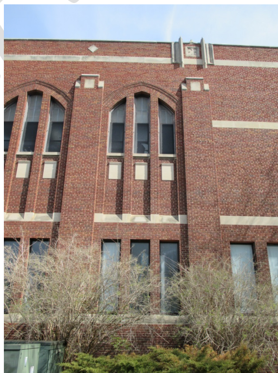
South Elevation – 1930 Wing (2014)
