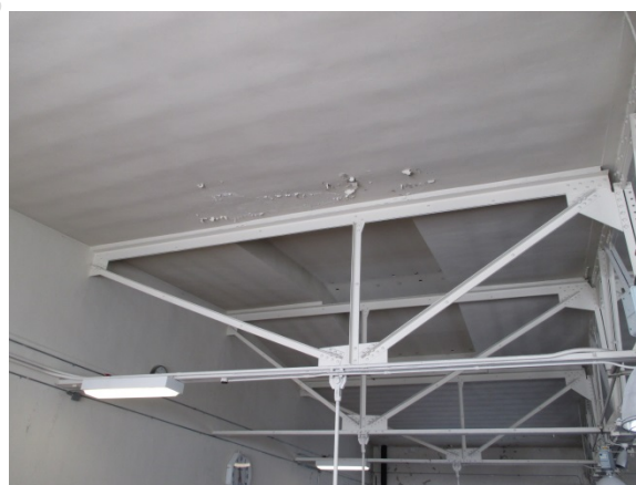
1916 Gymnasium Roof Structure (2014)
