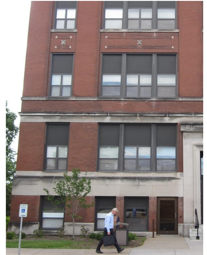
UW-Stout Harvey Hall – Prior to Renovation
