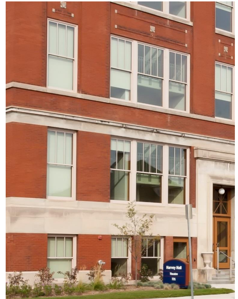
UW-Stout Harvey Hall – Completion
