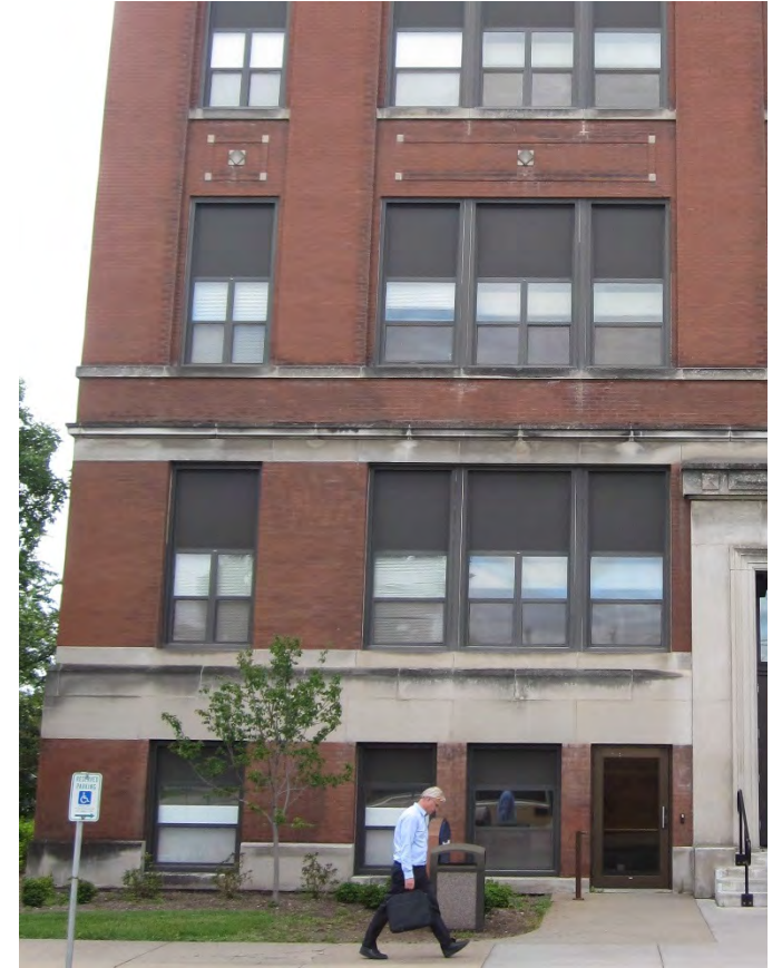
UW-Stout Harvey Hall – Prior to Renovation
