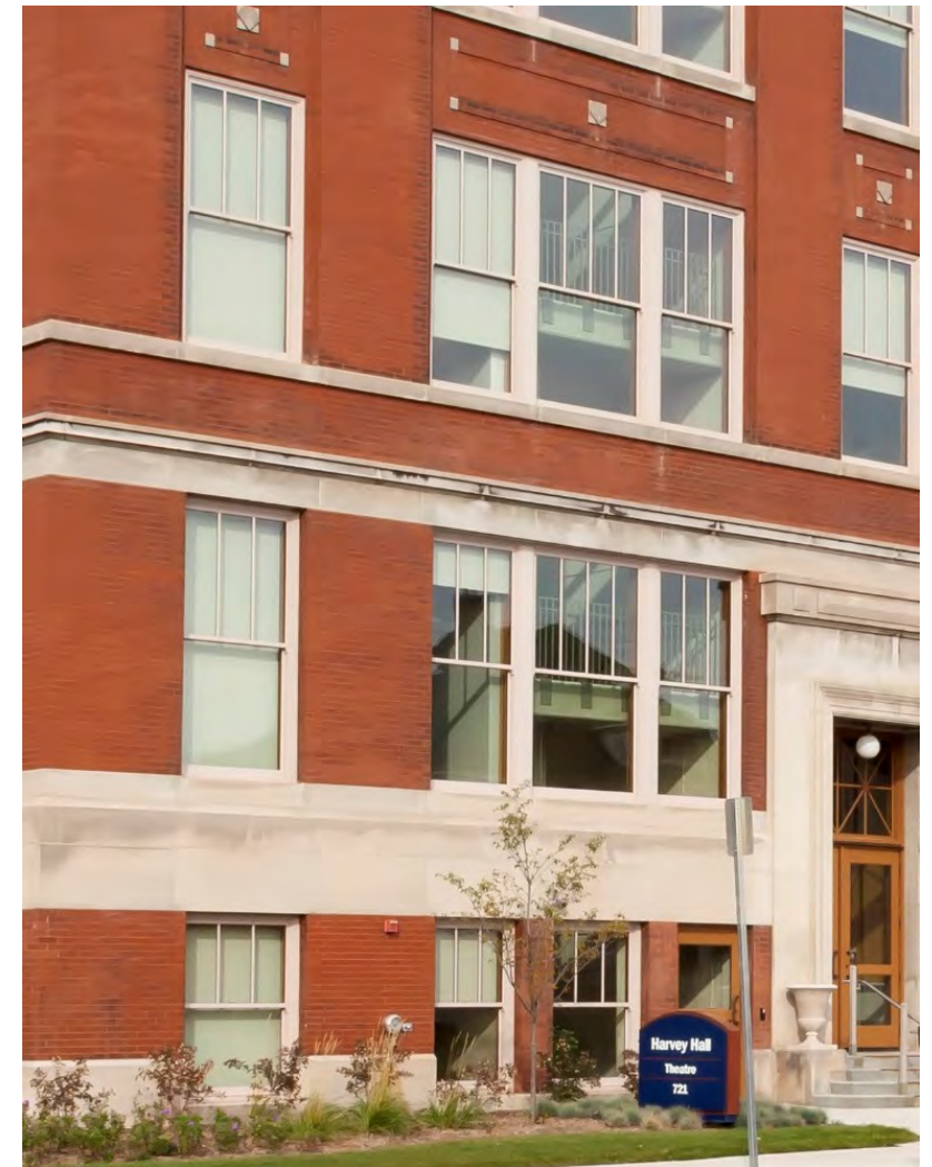
UW-Stout Harvey Hall – Completion
