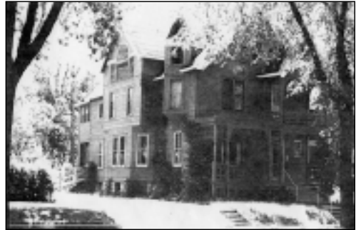
Figure 1. 1328 State Street - 1984 (Photo taken for the Intensive Survey)
