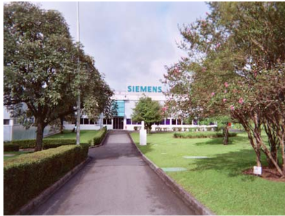
Figure 3. View of the main Siemens plant
