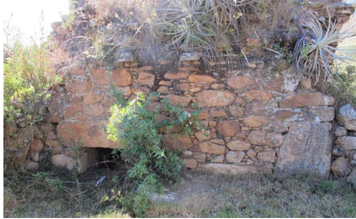
Figure 11. Lintel stone and cornerstone of chullpa .
