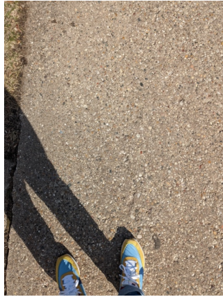
Figure 4. Sidewalk outside of original distribution location
